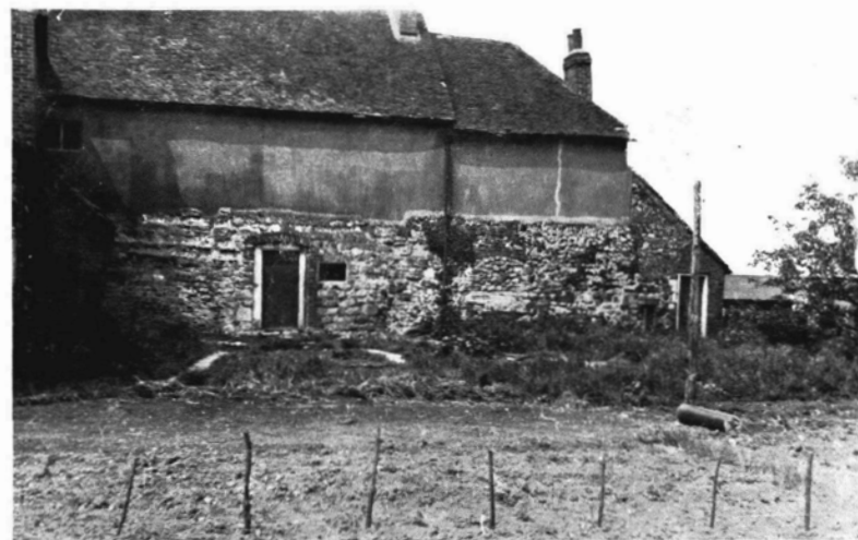
B. East wall of cottage showing medieval masonry and blocked doorway.
